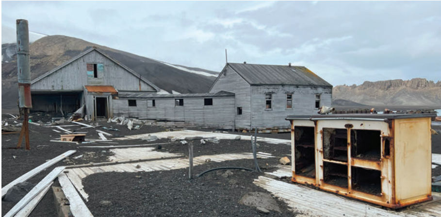
Plate 170. The remains of Station B, Deception Island, February 2024. A cooker unit stands on the site of the former cookhouse, with the main accommodation building in the background.
